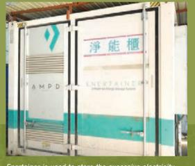
Enertainer is used to store the excessive electricity, mainly powering the tower cranes.
